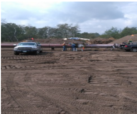
SF15 Complete weld - Inspection pass
