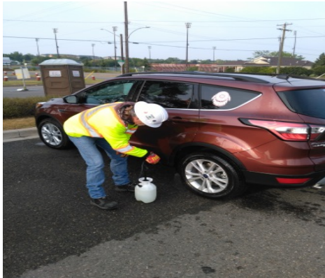
SF15 - Cleaning after sandblasting and coating - Brandon Coop Carwash
