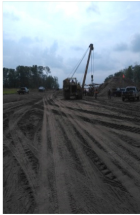
Side boom crossing roadway to unload truck
